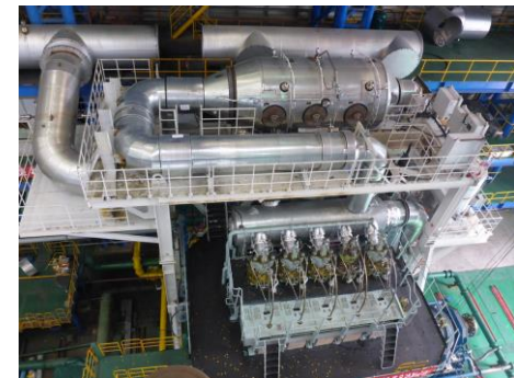
SCR-installation on WinGD field test vessel
